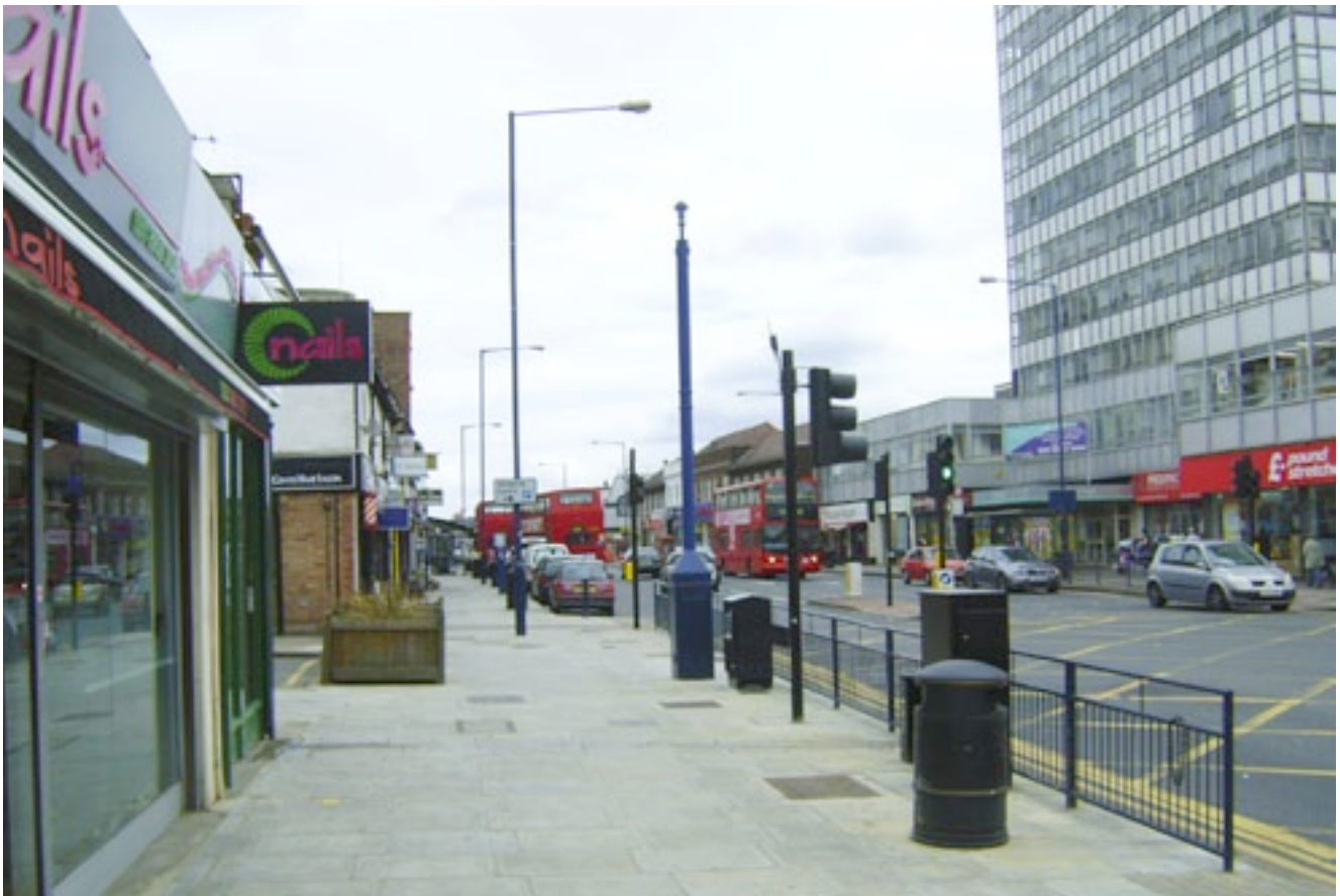
Existing high street environment within part of the Central Zone near Premier House
