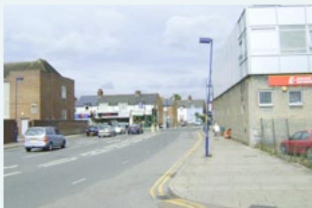
Existing access to the Broadwalk Shopping Centre
